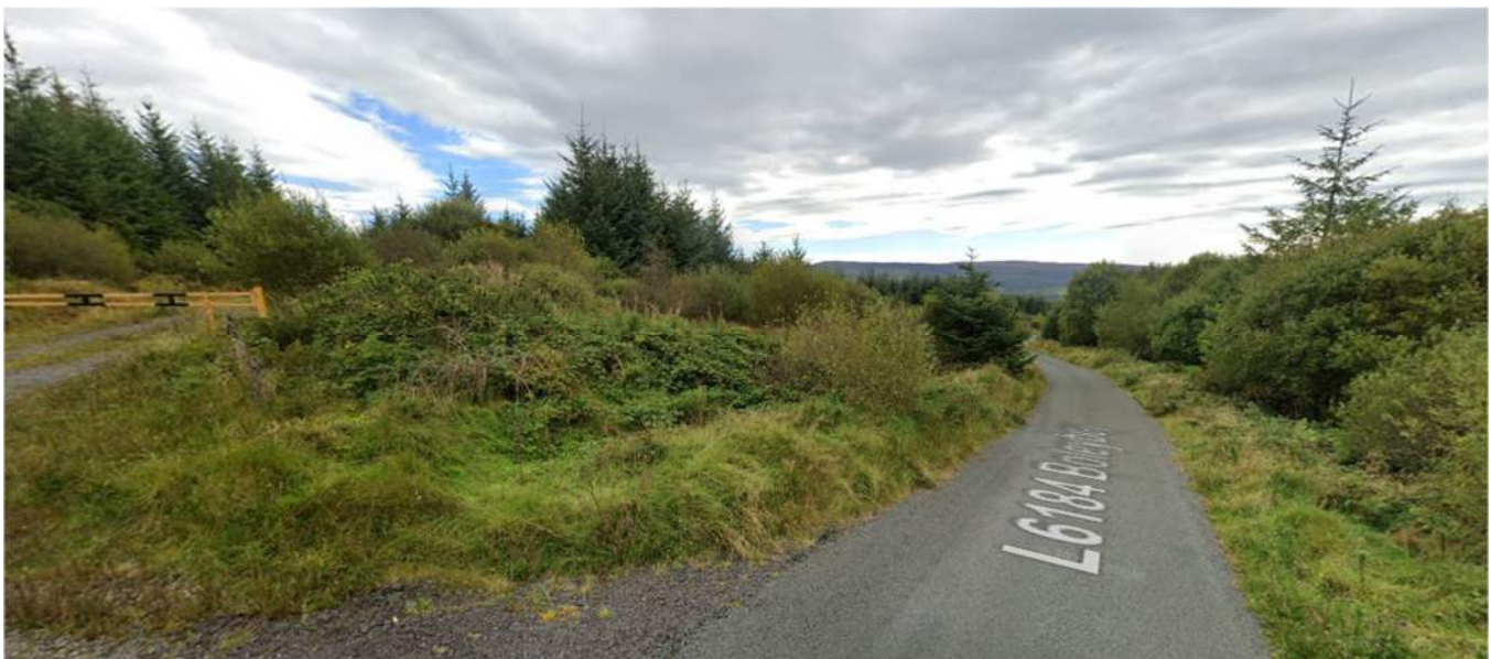
Figure 17: Road alignment from access to Borrow Pit 2 in a southern direction
