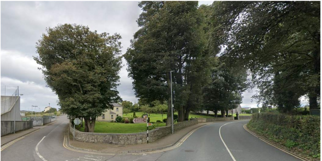
Figure 11: Existing boundary treatment in front of Parochial House and St. Clare's Church
